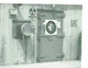
15. Entrance to the designated NHMFL bunker at Los Alamos that is used for explosive flux compression shots. The bunker contains full life-support systems.
