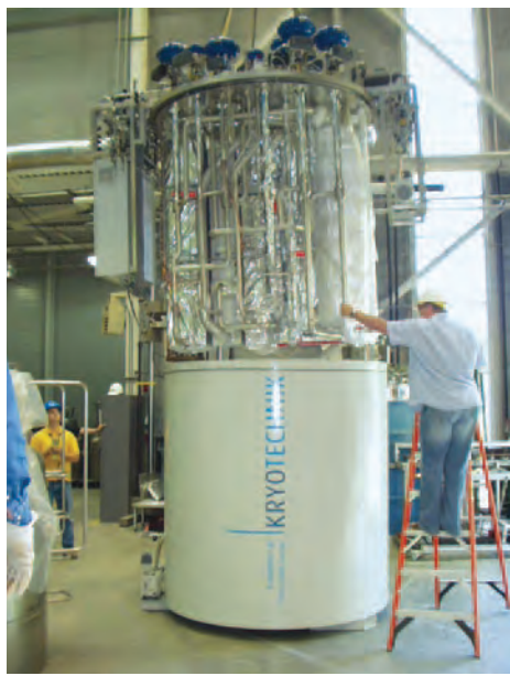
FIGURE 25. Installation of the helium liquefier in cell 16 of the Magnet Lab.
