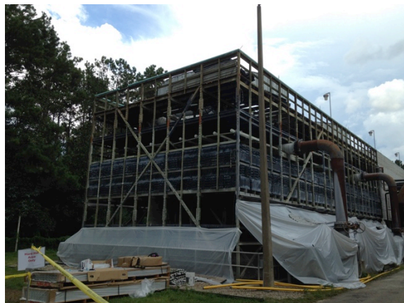
Figure 7: MagLab cooling towers undergoing renovation.
