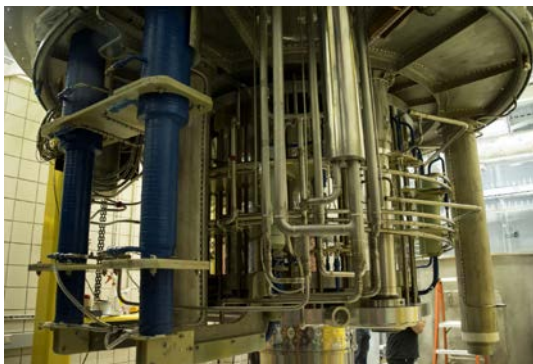
Figure 18: SCH Cold Mass, encircled by Plumbing for Liquid Helium, with the HTS Current Leads, coated in blue insulation, supported by the Top Plate of the Cryostat.
