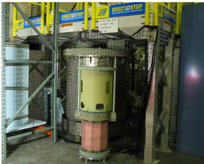
Figure 1: The new Duplex magnet sitting on the floor in front of the duplex magnet cryostat is housed in building 294 and will allow routine pulses up to 75 tesla for users in 2017.
