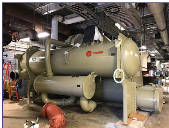
Figure 2.b.1: The first 7 MW (2,000 ton) chiller being installed.
