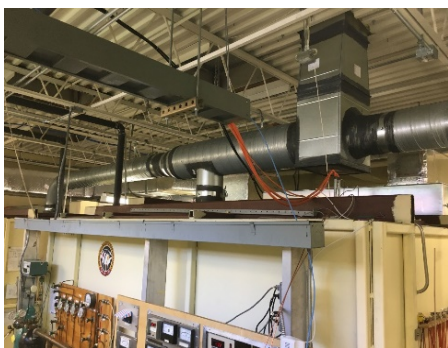
Figure 2.b.12: New helium exhaust ducts installed above the three "bays" (magnet stations).
