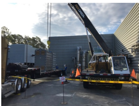
Figure 6: New magnet cooling water heat exchanger being delivered outside the DC Field Facility plant.
